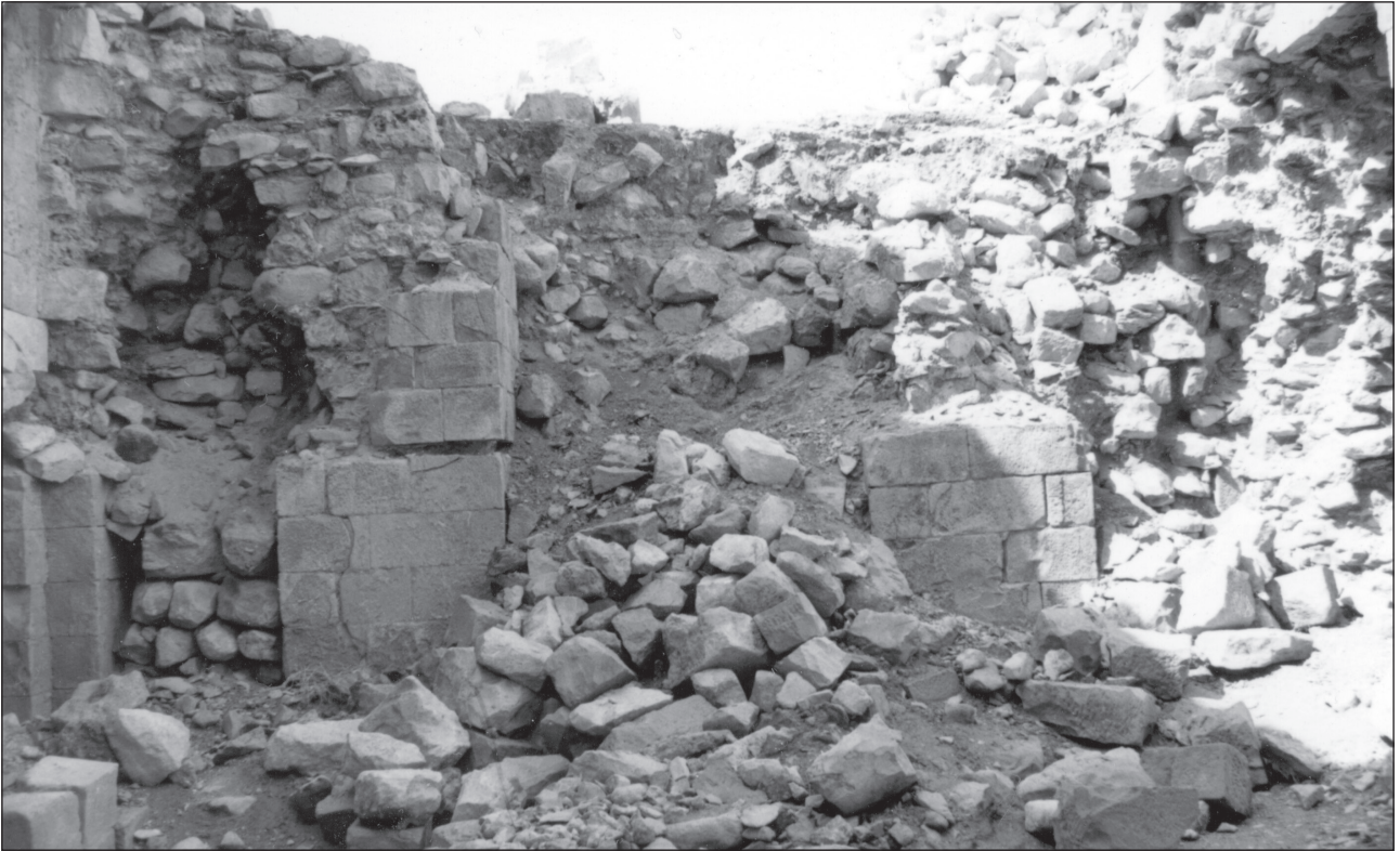
5. Palace qa'ah at Shawbak, entrance to the grand iwan (blocked with rubble), view north-west from the durqa'ah .
